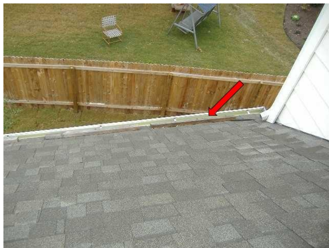
1. Roofer walk boards are still present. Nail holes should be sealed after removal.
