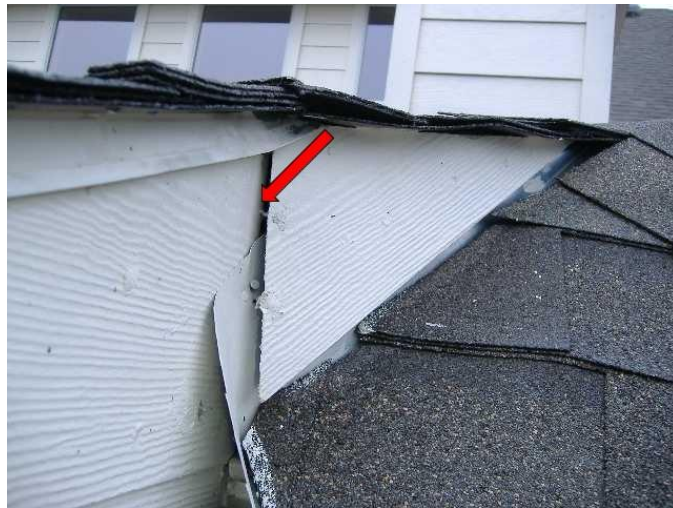
1. Roofer walk boards are still present. Nail holes should be sealed after removal.
